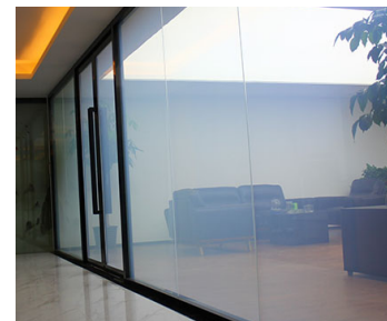
Figure 1 : (Left) Visual appearance of a privacy active glazing in the transparent and scattering mode. (Right) Residual haze in angle in the transparent state.
